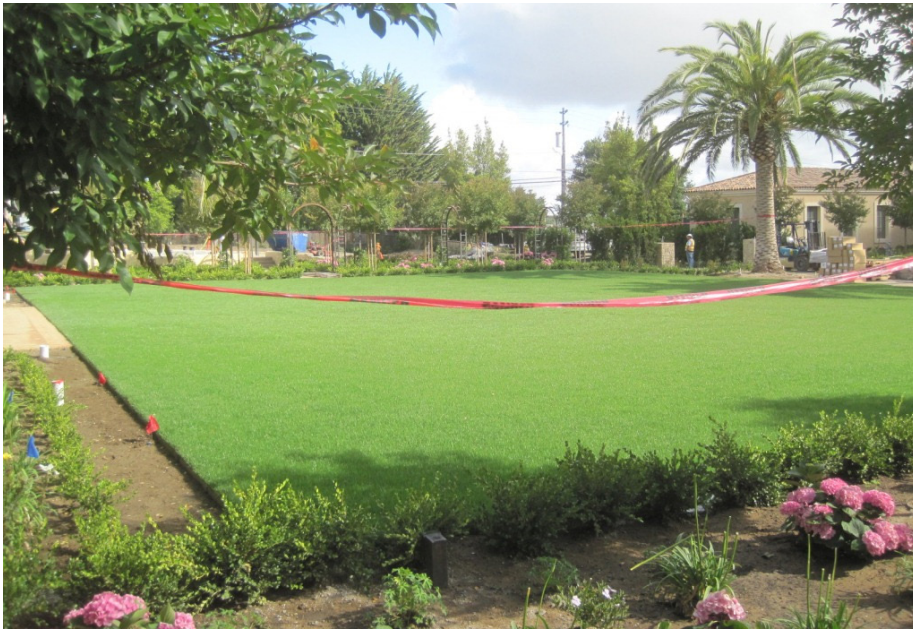
Sod is installed to provide permanent vegetation and erosion control.
