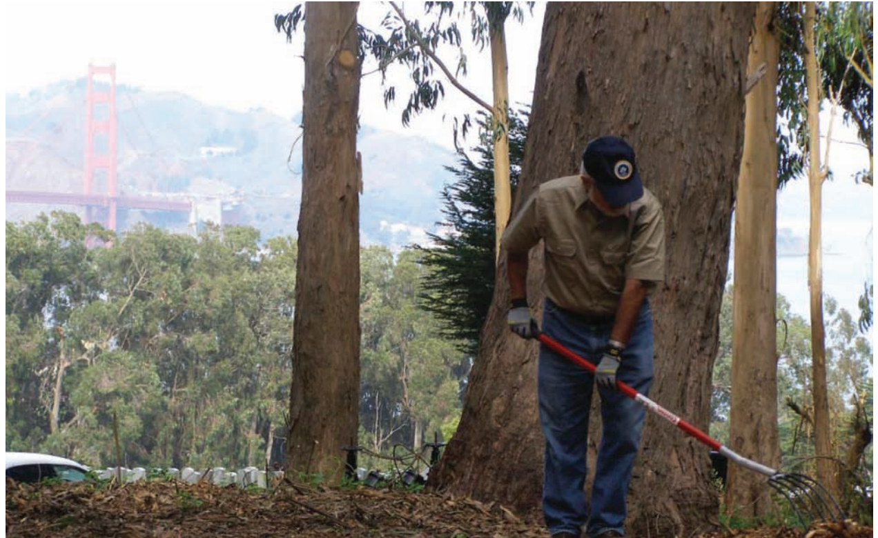
Wood mulch is applied to landscaping to reduce erosion and to help with vegetation establishment.
