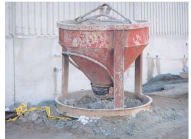
Wastes from concrete curing are not contained, and are open to contact with runoff.
