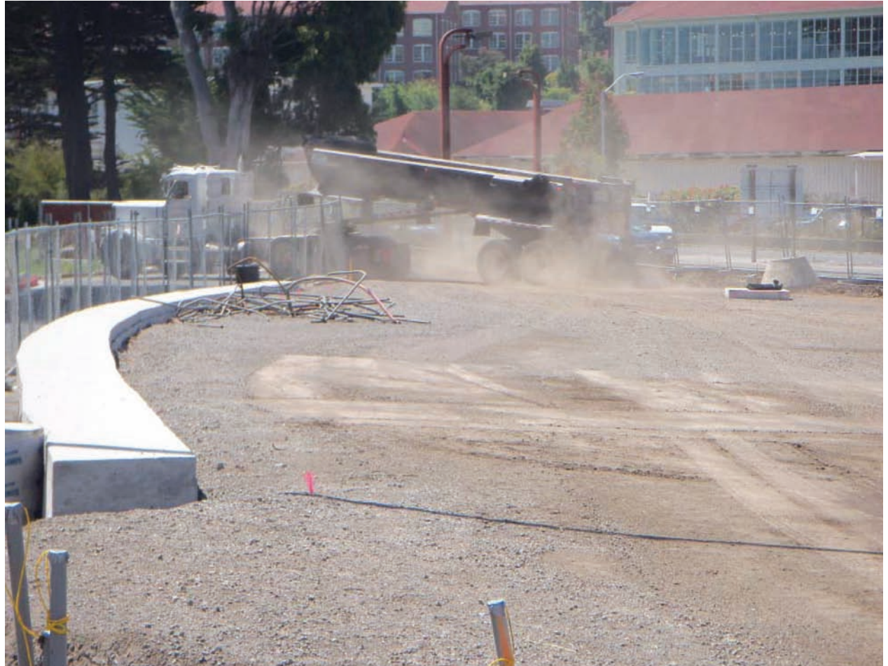
In order to reduce the dust generated by delivery trucks, water should be applied to all disturbed areas.
