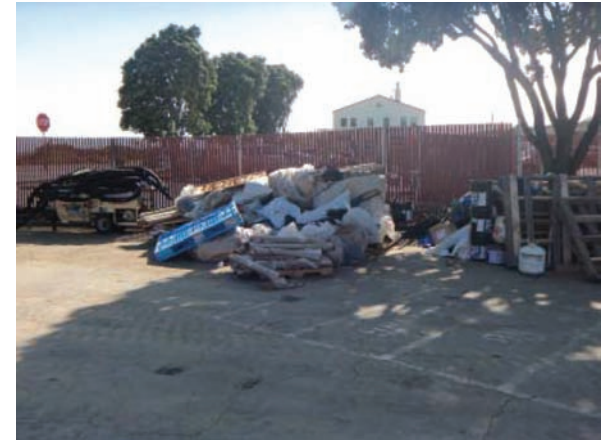
There are no dumpsters, containers or diversion structures to stop stormwater runoff from coming in contact with this construction litter and debris.
