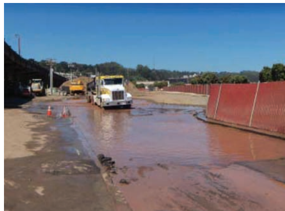
Construction area without a tire wash.
