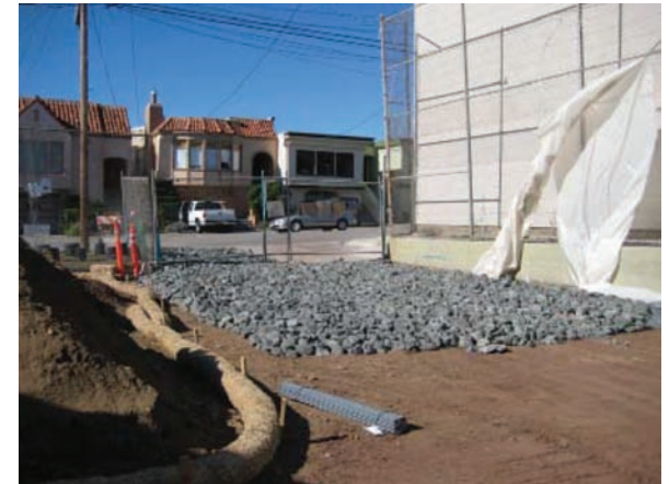
A gravel construction access is properly installed at the site entrance.
