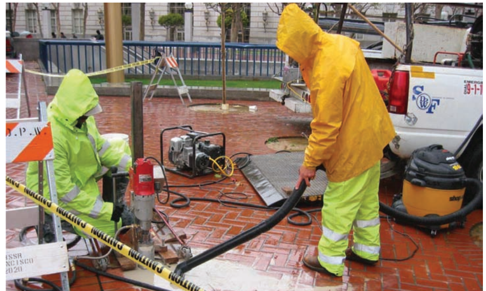
Workers vacuum liquid waste from drilling activities.
